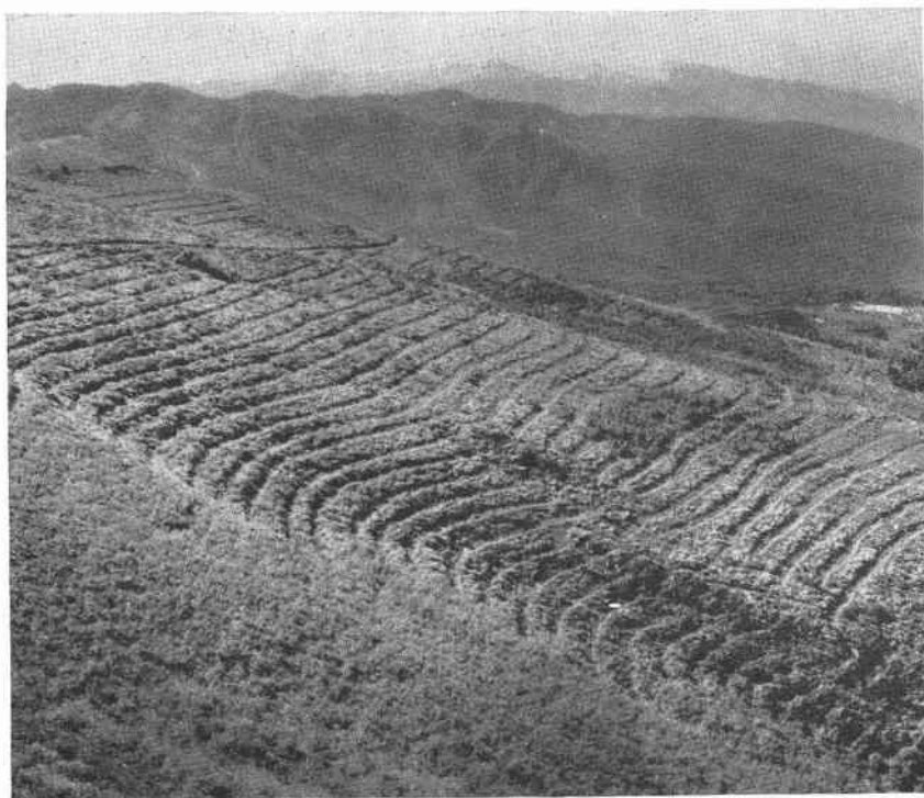
Contour trenching and reseeded to repair a damaged watershed that had been a frequent source of disastrous floods. Davis County, Utah.
