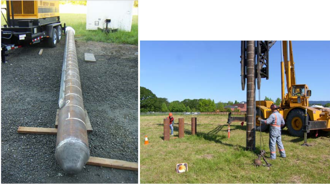
Figure 3-15 Installation of Baseline Pile (I-1)
