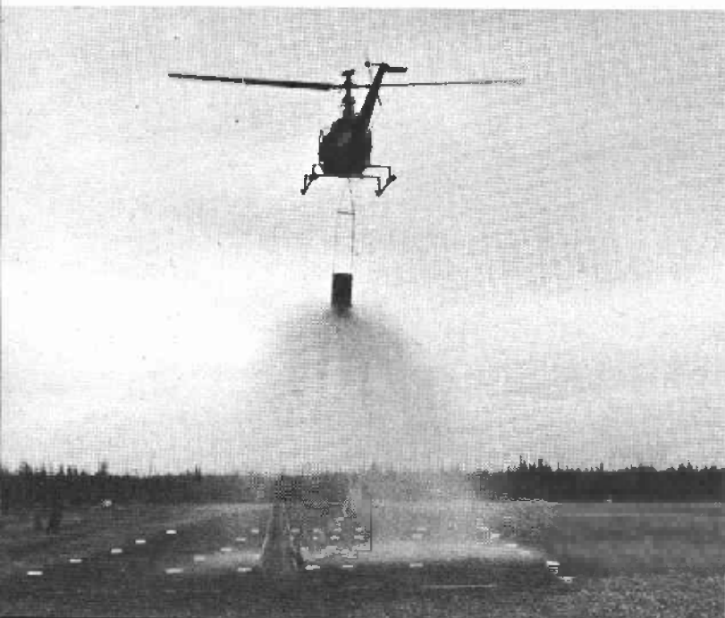
Helicopter waterdropping calibration test carried on through cooperation with the Bureau of Land Management and the U.S. Army at Ft. Wainwright, Alaska.
