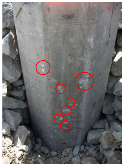
(b) Pock-marks, evidence of point load
