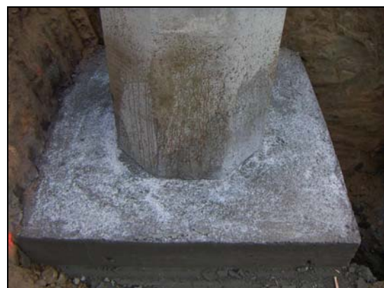
(l) Just after removing formworks
