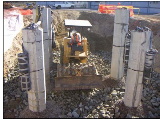
(j) Compacting with vibro-roller
