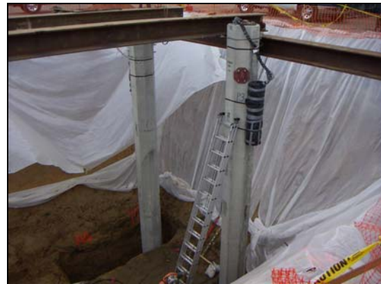
(h) Installed piles
