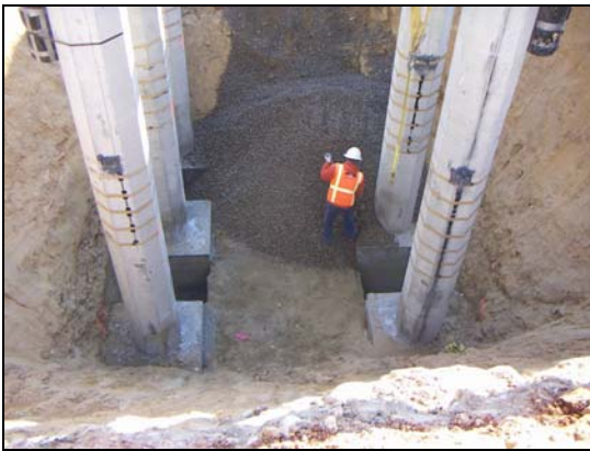
(c) Backfilling bottom of the pit with gravel
