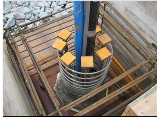
(h) Finish installation of the dowels
