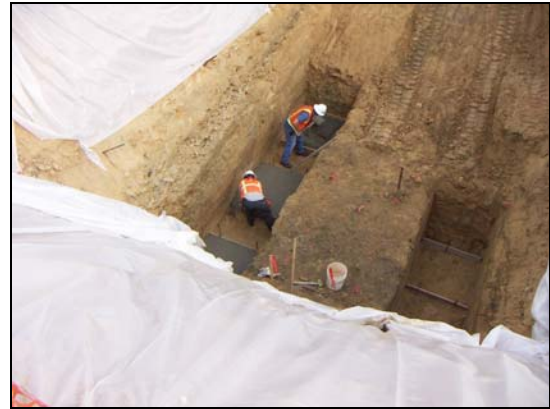
(b) Building concrete slab at the bottom
