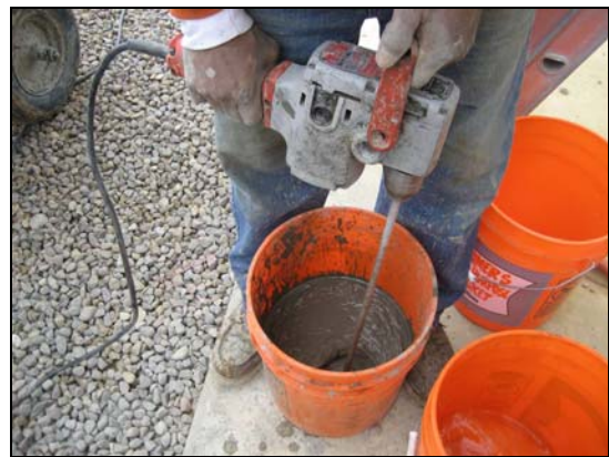
(f) Mixing grout material
