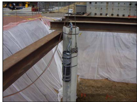
(f) Installed pile fixed to the beam
