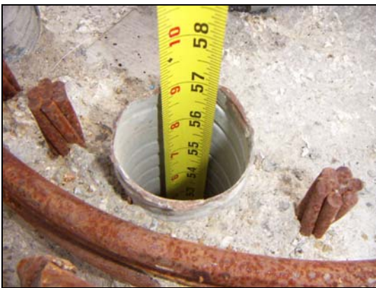
(e) Measuring depth of the dowel tube
