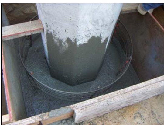
(k) Pouring concrete to the footing
