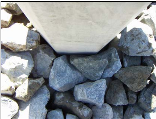
(k) Gap between the pile and the rockfill
