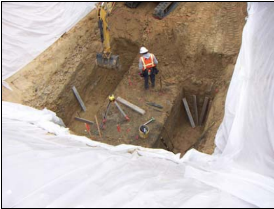
(a) Excavating trench for footing
