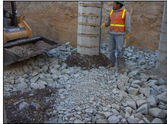
(h) Placing gravel around the sensor
