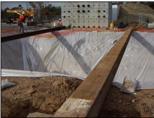
(c) Placing steel beam fixing pile tops
