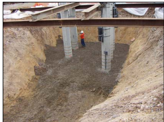
(f) Finish the first stage of backfilling
