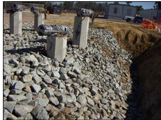
(l) Finish backfilling
