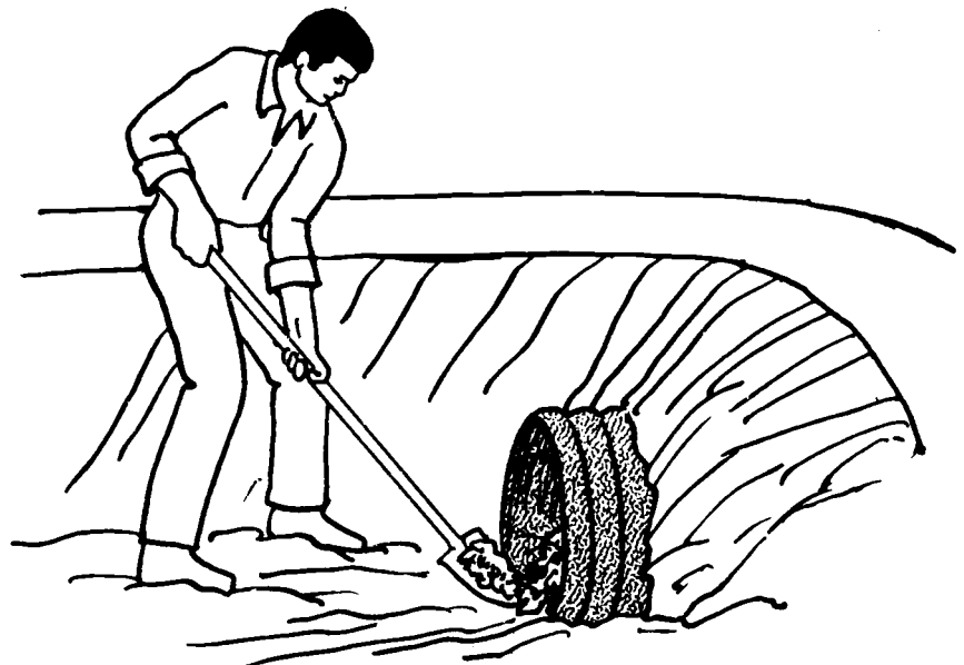
Figure 1.—A hand shovel is all you need for some important maintenance work like culvert cleaning.
