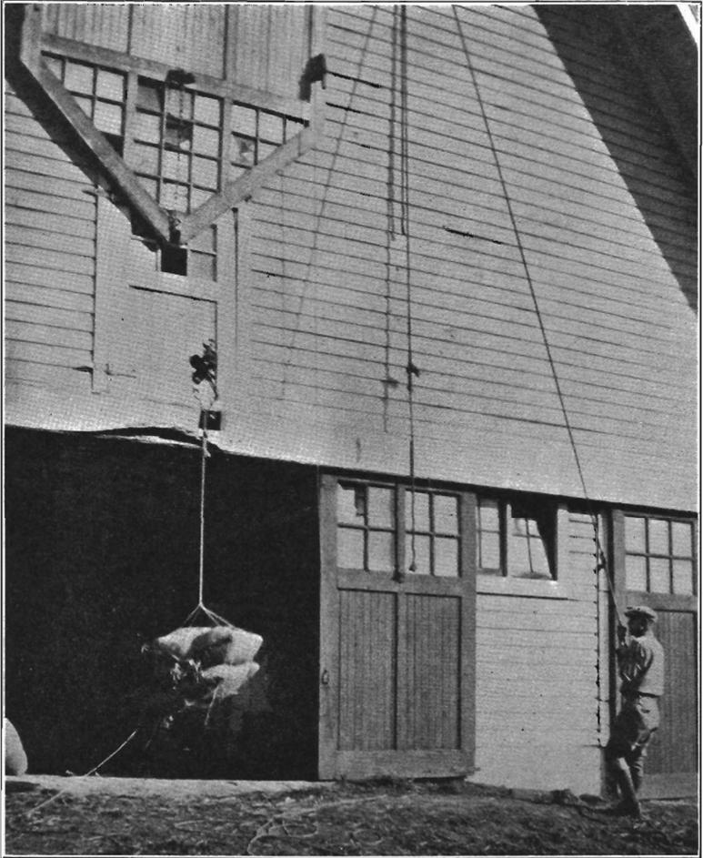
Fig. 7. Hoisting sacks of grain to be emptied into bins. Operator is pulling the control rope to engage the hoist clutch. A hay sling trip is used to drop the sacks.
