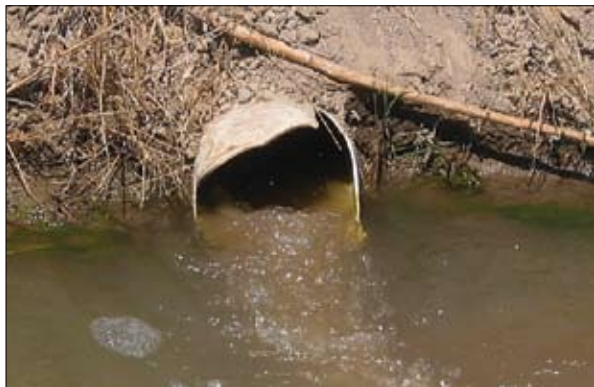
Figure 4. Runoff from an onion field with no erosion protection.
