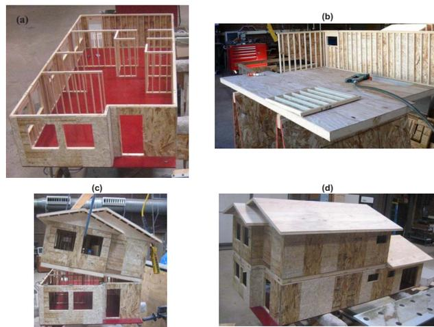
**Fig. 1.** Construction sequence (a) assemble first floor walls; (b) assemble second floor; (c) lower second floor on top of first floor; and (d) completed structure
