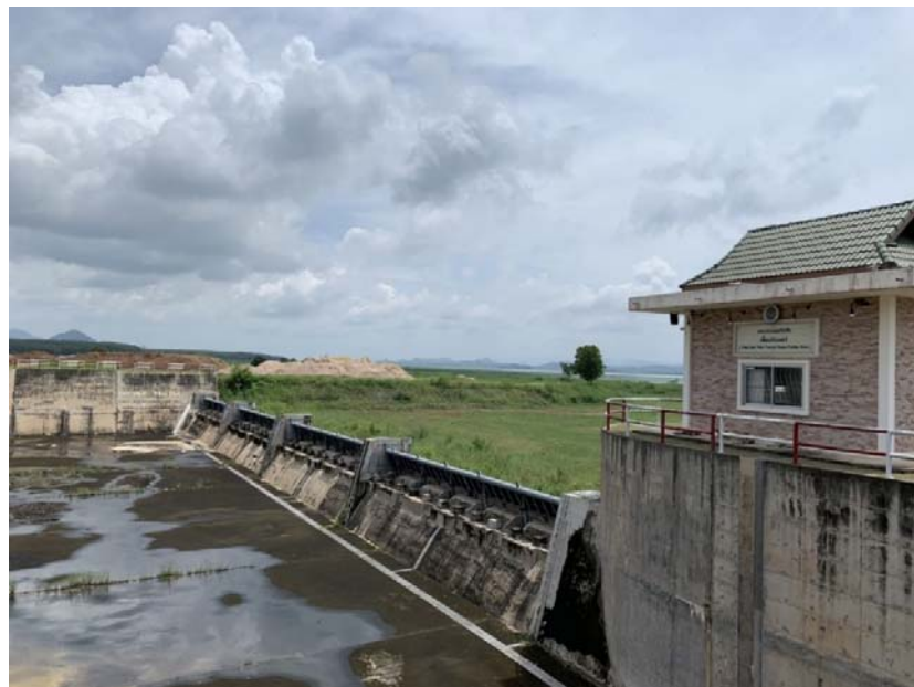
Figure 36. Flap Gate Weir and Control Room
