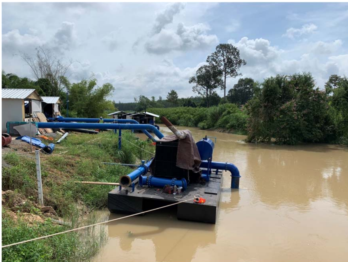
Figure 46. Khlong Saphan Temporary Pumping Station
