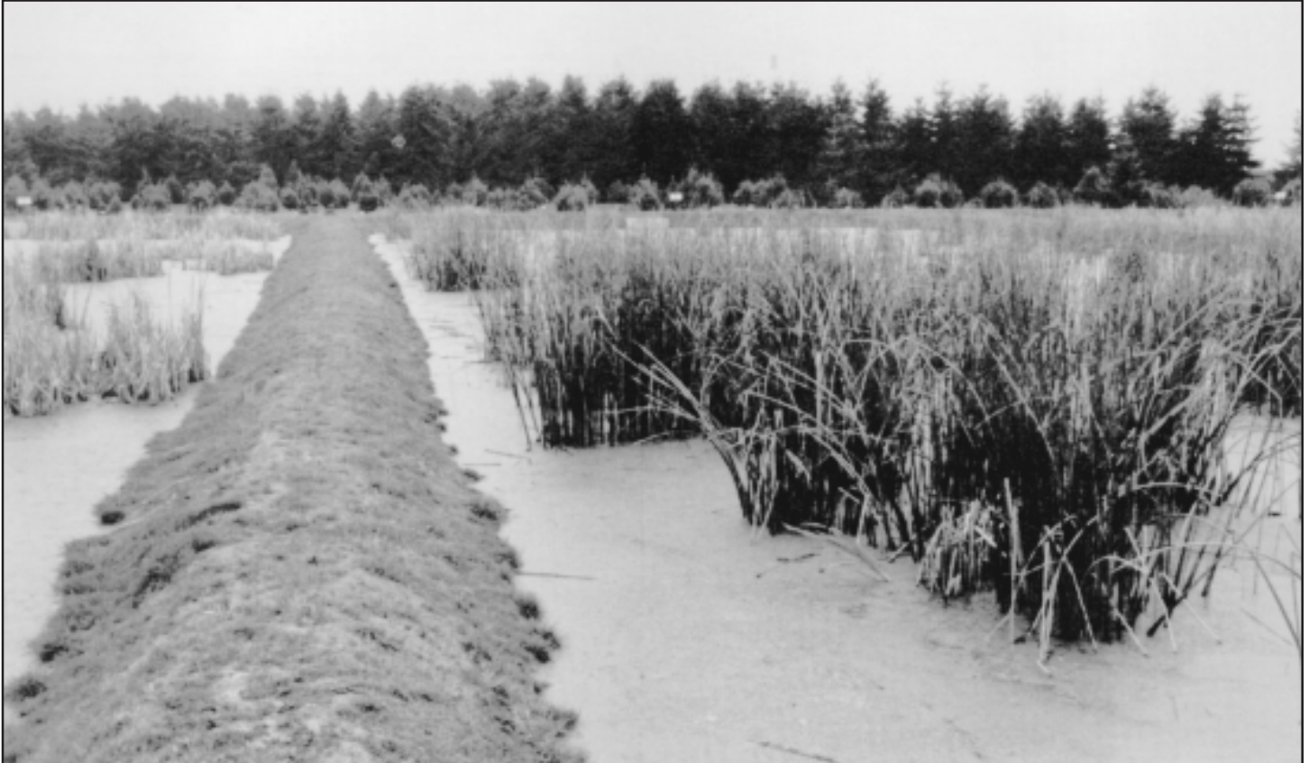
Figure 2.—Constructed wetlands commonly use earthen dikes to control flow of effluent and treatment time.
