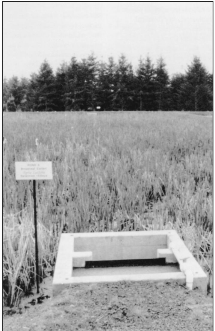
Figure 1.—Concrete control boxes (foreground) regulate flow rate and water depth in constructed wetlands
