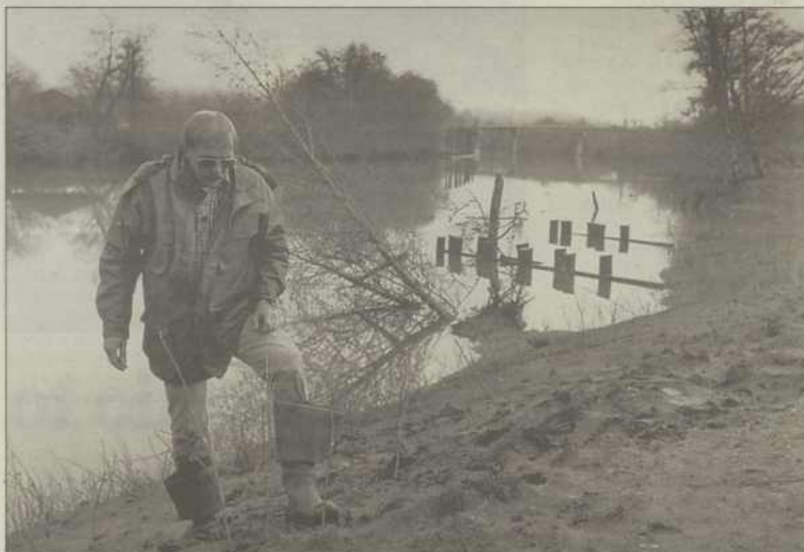
Oregon State University marine extension agent Paul Heikkila plants willow trees to stabilize the bank of the Coquille River, a prime salmon stream on Oregon's South Coast. Many landowners in the area are working to improve salmon habitat, says Heikkila.
