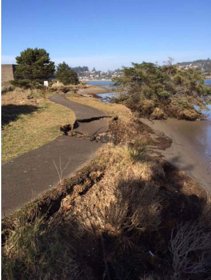
Figure 4.6: View to the north in the Reference area (January 26, 2013), showing collapsed banks with vertical scarps and additional section of collapsed asphalt due to continued rapid erosion.
