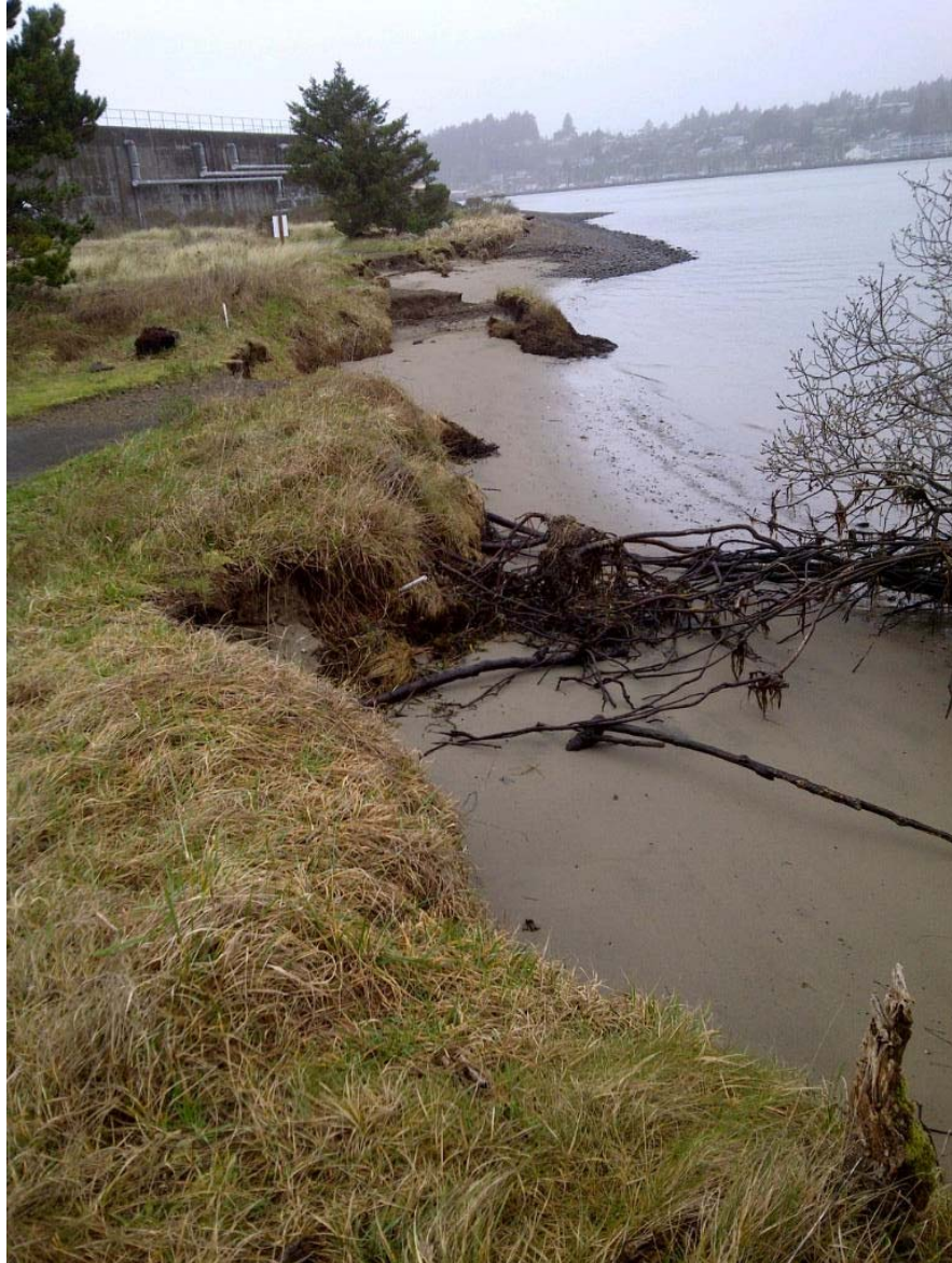
Figure 4.3: View of eroded section of HMSC nature trail, February 14, 2014. The terminus of the 2011 dynamic revetment is seen in the upper center of the photo, and the offset caused by shoreline erosion is clearly visible.
