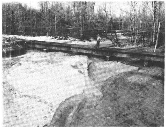
Figure 3.—This railroad bridge had to be raised three times at a cost of $300,000 because sand eroding from the hill-sides repeatedly choked the stream channel.
