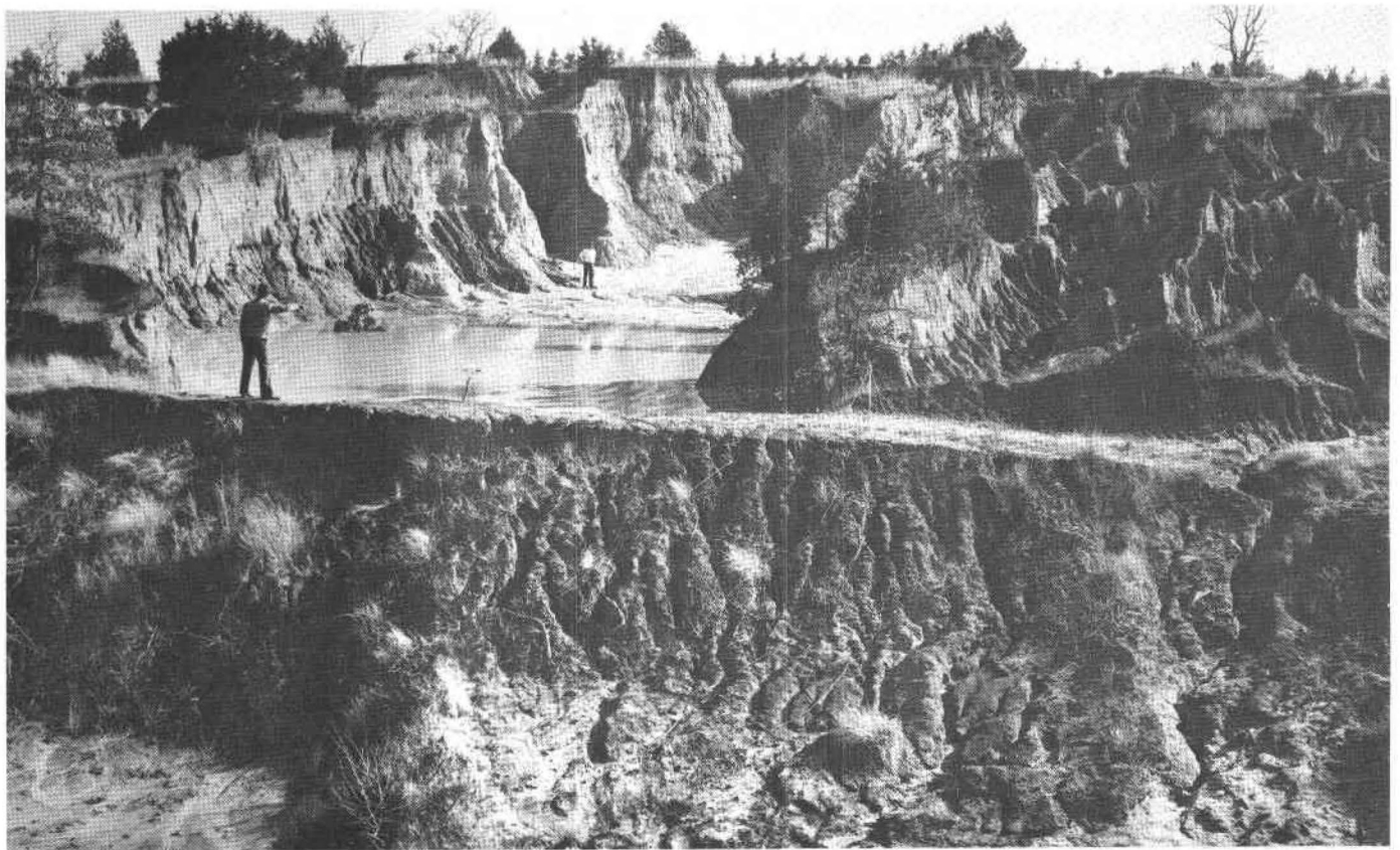
Figure 11.—A "gully plug" was constructed to prevent the land below from sedimentation. Planting trees and lovegrass above the gully plug stabilizes the soil within 10 years.
