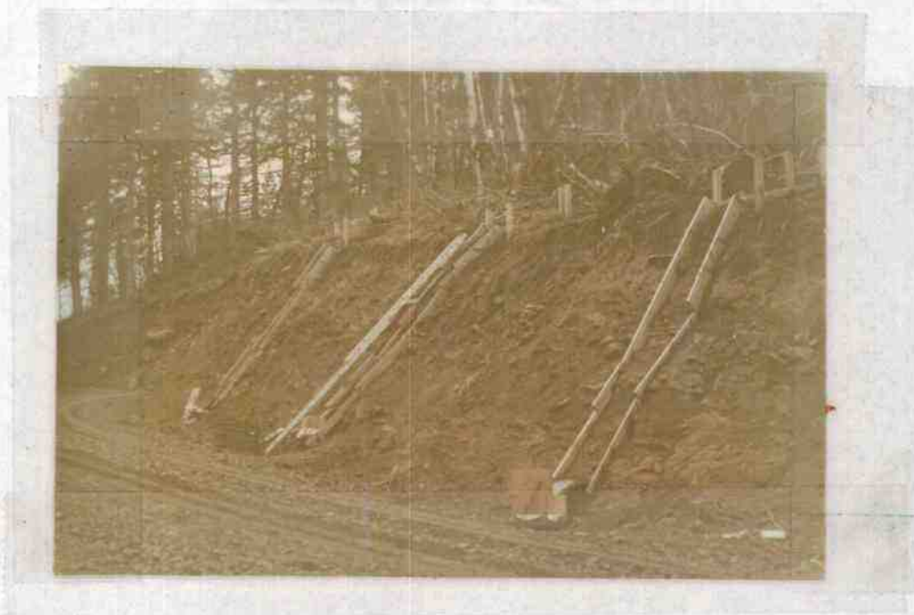
Figure 4. Photograph of the cut slope and three cut slope plots.
