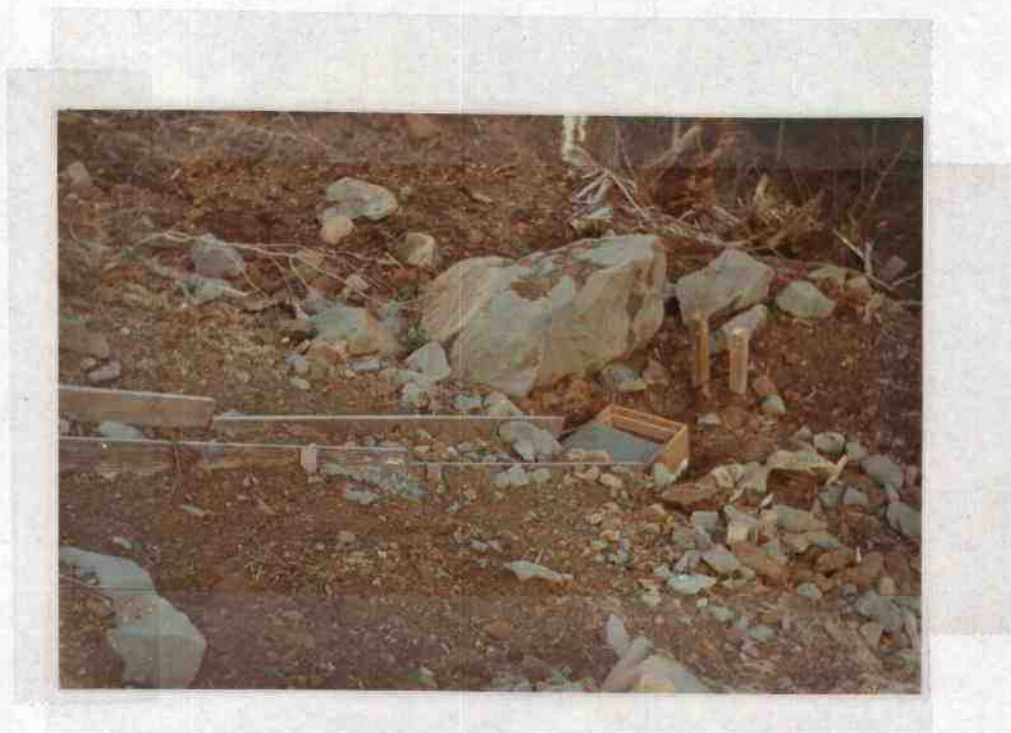
Figure 3. Photograph of downslope view of fill slope plot number 4.
