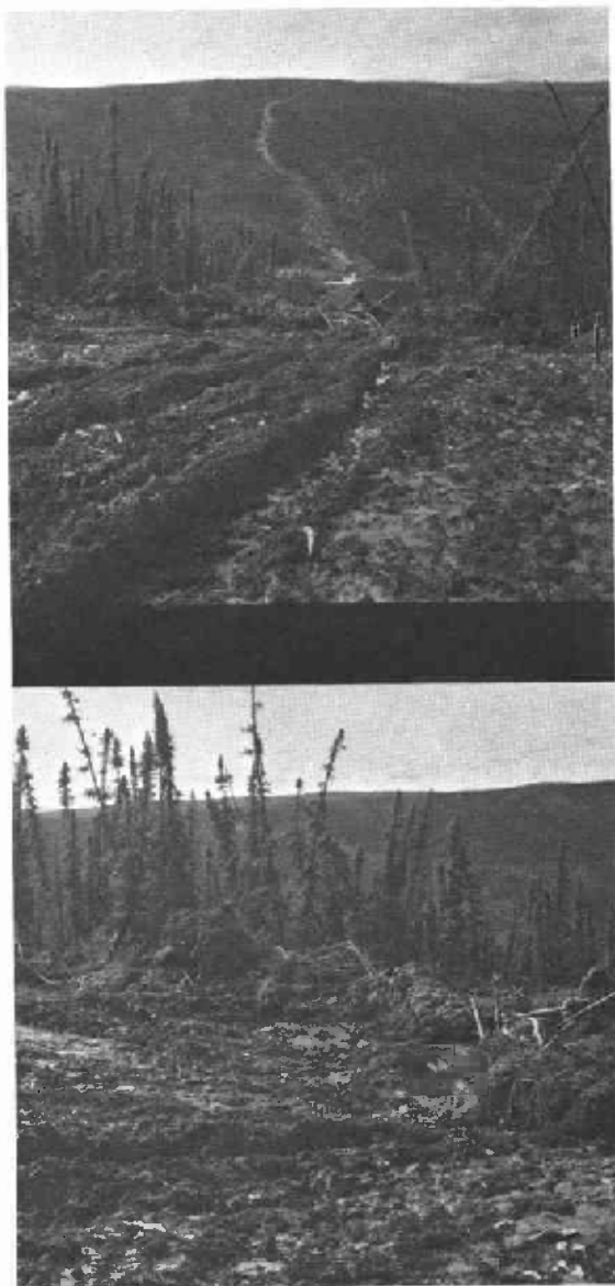
A consequence of fireline construction in areas of permafrost is thawing and cancerlike erosion. Permafrost covers 90 percent of interior Alaska.
