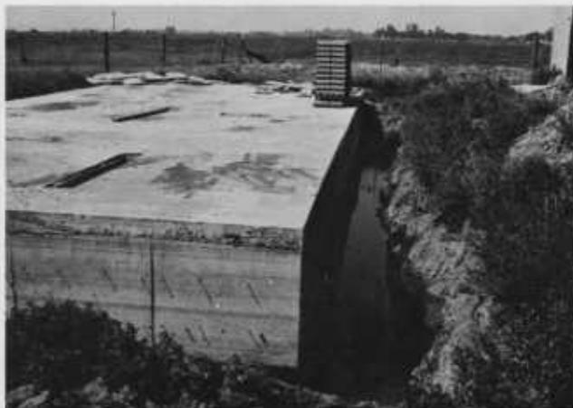
Figure 13. High water table during rainy season can cause concrete liquid tanks to rise out of the ground when empty unless tank is anchored properly.
