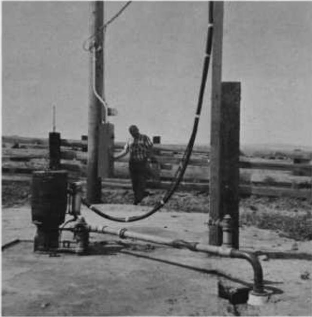
Figure 6. An electric-powered chopper-type pump installed on liquid holding tank for distribution by the sprinkler method. Pump has a built-in agitation system. An electric fence is used around the tank area to keep animals away from the pump and tank opening.
