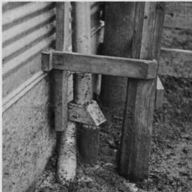
Figure 14. Gutters and downspouts on eaves can prevent hundreds of gallons of excess rainwater from entering manure tanks.
