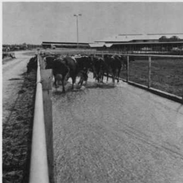
Figure 8. A flush-down manure removal system.
