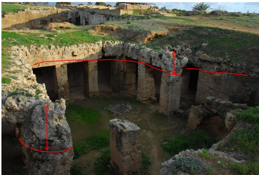
Figure 3-28 Kafkalla cap on MIS 5 (5c and 5d) aeolianite deposits west of Pafos. Tombs (appr. 2000 BP) are carved in the softer calcarenite below, taking advantage of the kafkalla cap as a stable roof.
