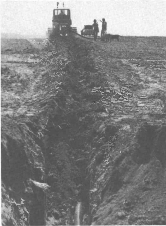
Fig. 4. Appreciable disturbance of the soil above the tube occurs with this method. Under the right soil conditions, topsoil mixing into the "backfill" to maintain sustained high infiltration potential is appreciable.
