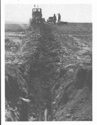
Fig. 4. Appreciable disturbance of the soil above the tube occurs with this method. Under the right soil conditions, topsoil mixing into the "backfill" to maintain sustained high infiltration potential is appreciable.
