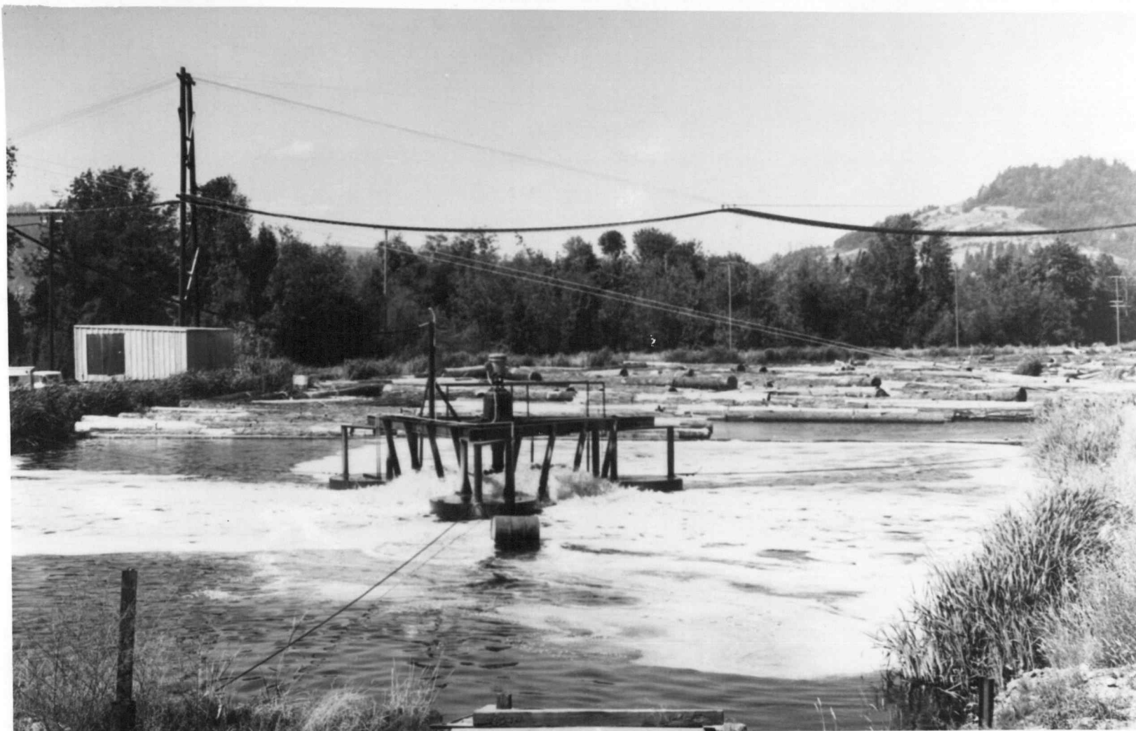
PLATE II 75 horsepower floating aerator churning air into Kraft mill effluent pond. Mixing is by a large propeller-like beater.
