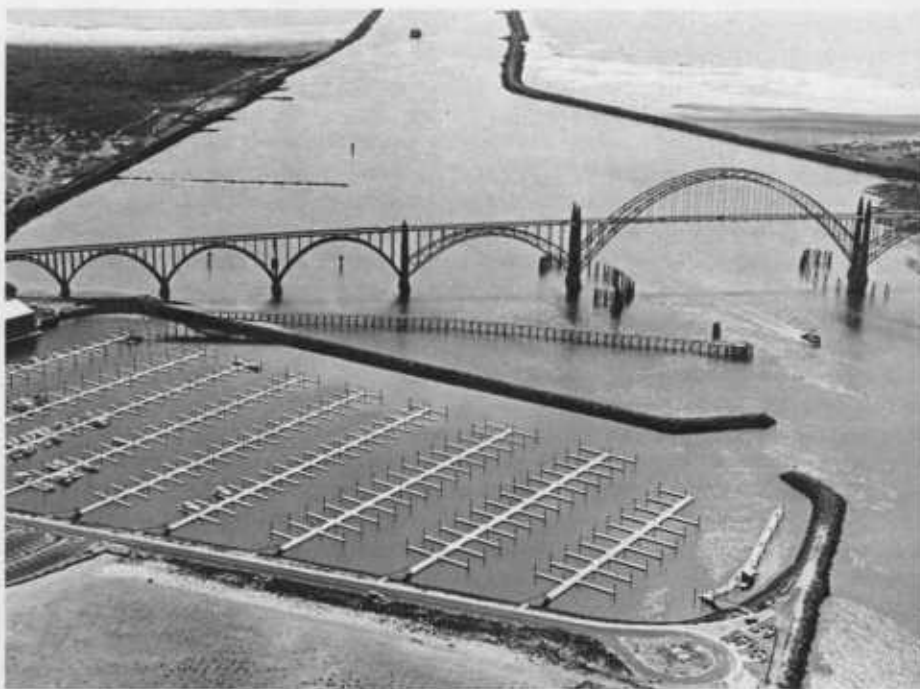
Major projects, such as this large marina, can require several years for planning, environmental assessment, and construction....
