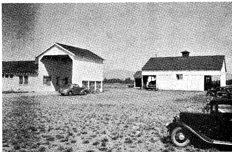
A modern flax plant showing covered drive over scales adjacent to office building and the deseeding building in the background.
