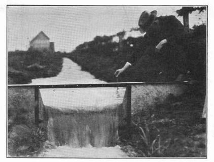
Figure 4. Weir measure showed up to 2 cubic feet per second. Discharge at the Brown Farm, Gervais, Oregon.
