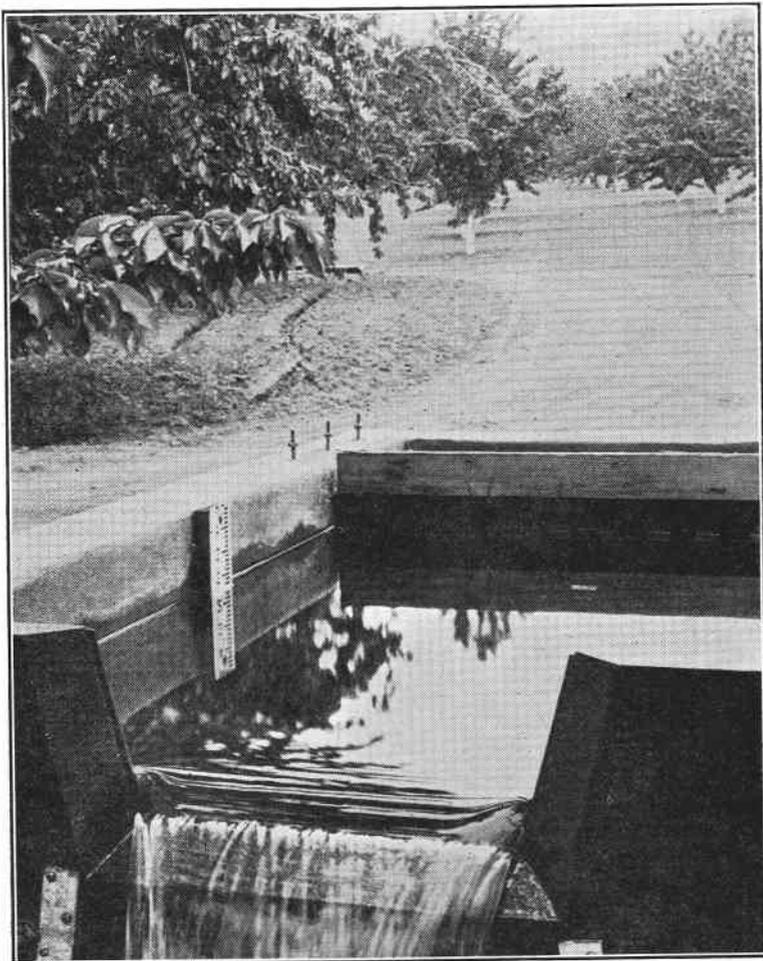
Figure 5. Ground water for irrigation; maximum lift 445 ft; discharge 175-230 gallons per minute. Cherry Hill Dist. Improvement Co., The Dalles. (Photograph by A. M. P.)
