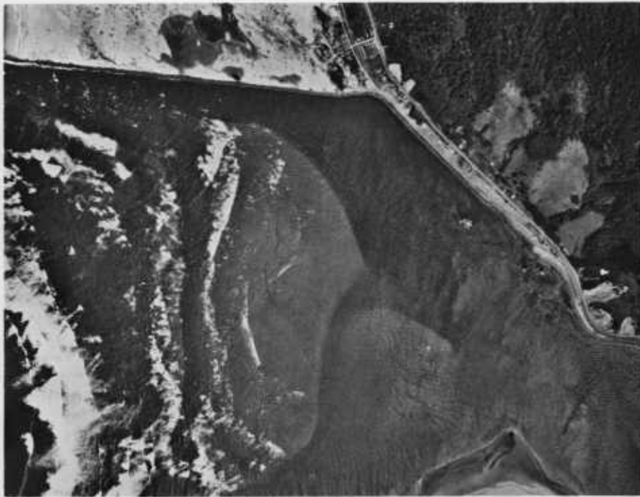
Figure 13.—For many years the entrance to Tillamook Bay was protected by a single jetty, on the north side of the channel. This jetty, in the upper left of this 1939 aerial photo, interrupted the littoral drift, accumulating sand to the north. Note also the rough water on the bar and to the south of the channel, with the single jetty installed.
