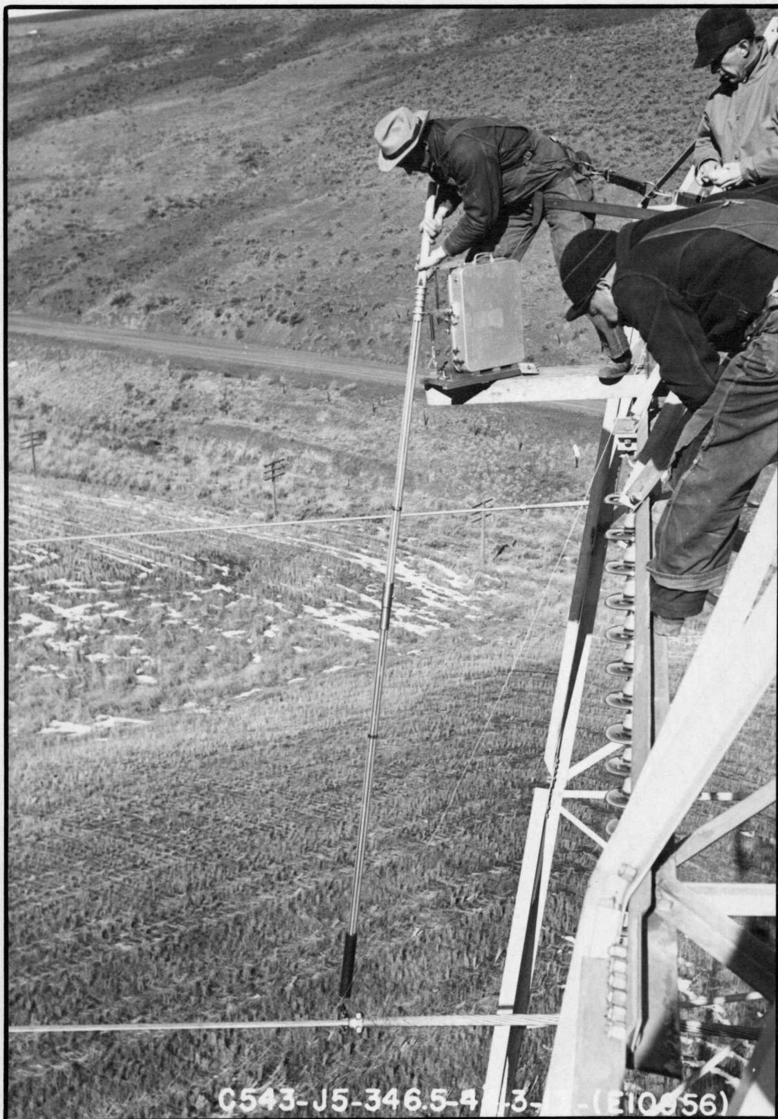
Figure 2. Installing a vibration recording unit.
