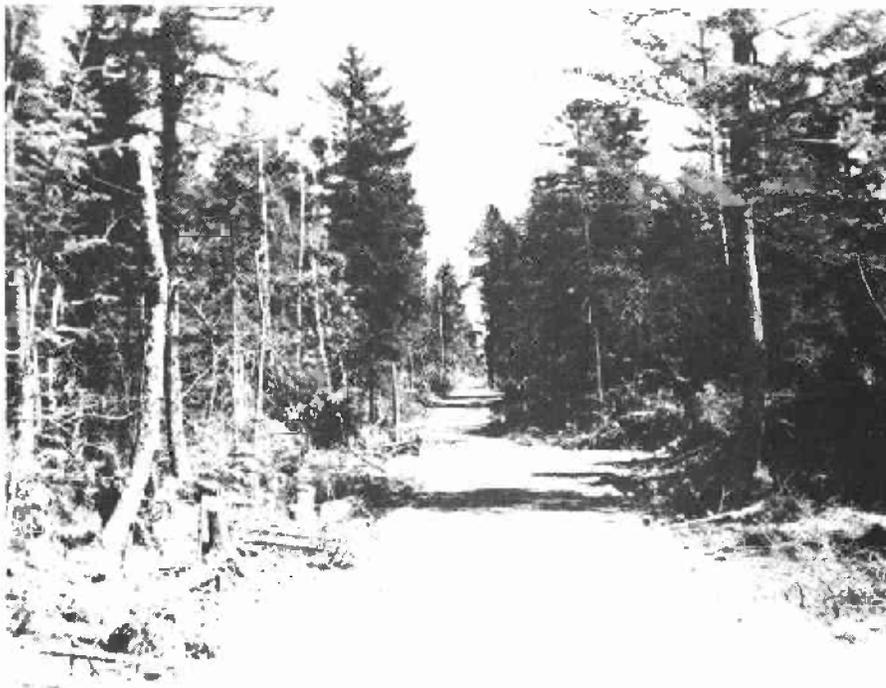
Figure 2.--Good alinement on a logging road in the same type of timber and terrain.
