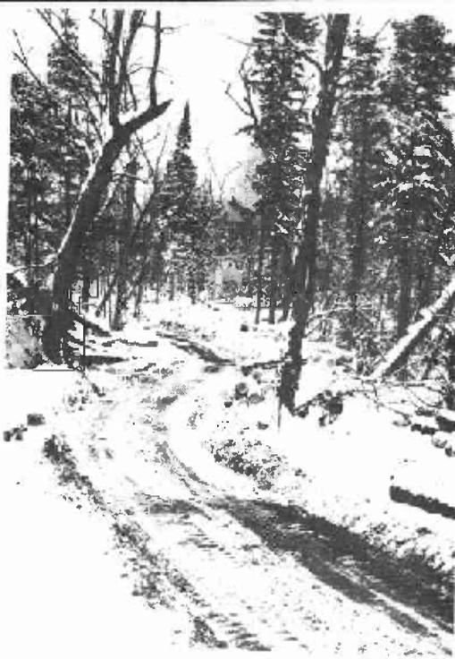
Figure 1.--Poor alinement on nearly level ground. A single flat curve could easily have been built. On some roads kinks of this kind have been observed where the road could have been straight.
