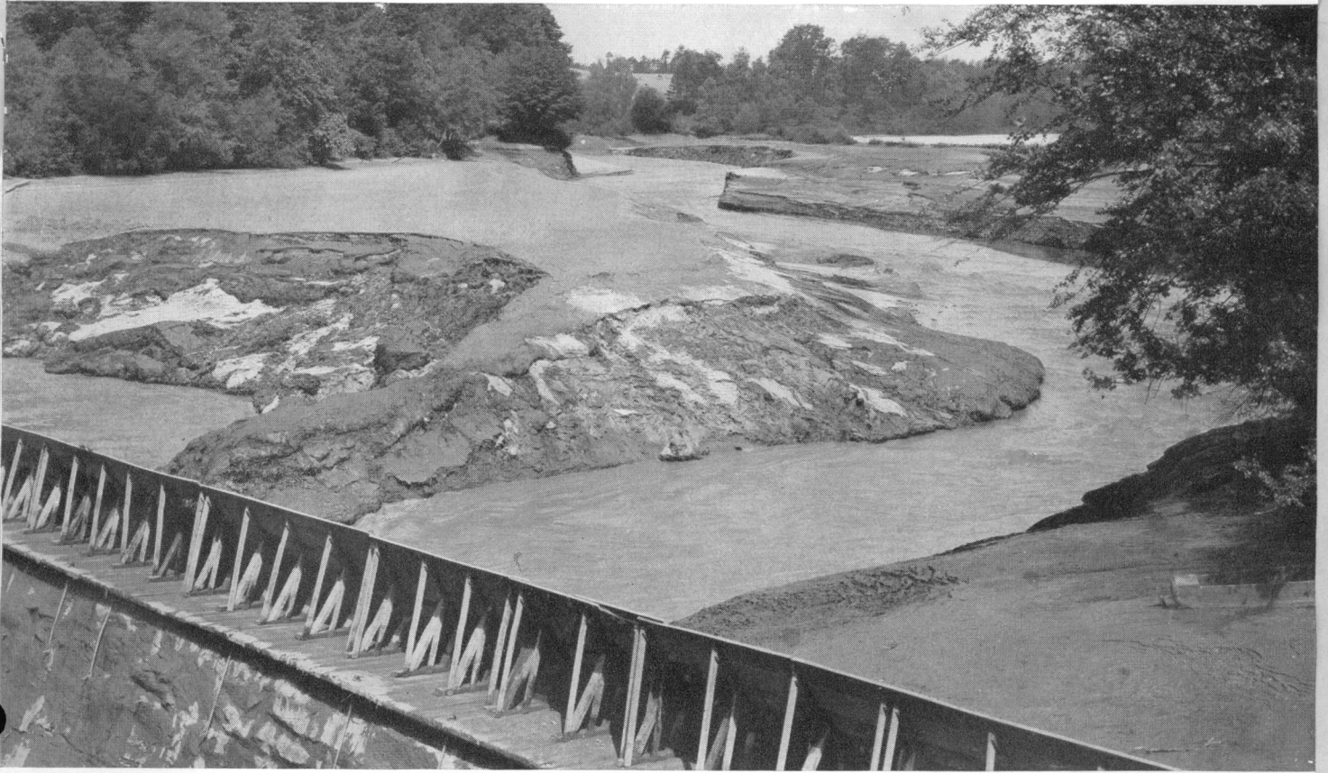
FIGURE 9.—Reservoirs filled quickly with silt and lost much of their storage capacity. Many Piedmont reservoirs filled in less than 30 years.
