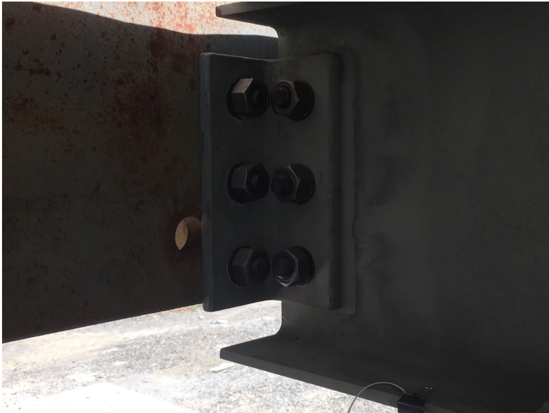
Figure 8: Ecoroof structural member double angel shear connection.
