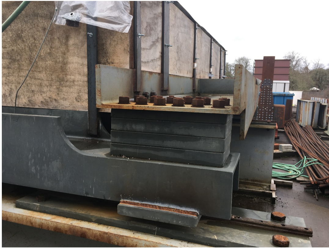
Figure A 9: Upslope Connection between W12x106 and W21x111, with Stacking Plates to Create Roof Slope
