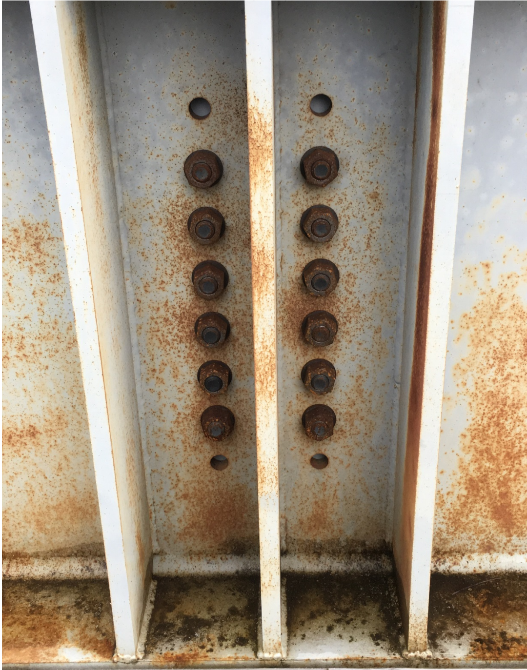
Figure A 1: Northwestern connection between W40x324 and W21x111 crossbeam.
