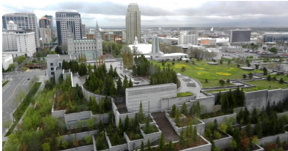
Figure 2: Latter-Day Saint Conference Center with Intensive Ecoroof, Salt Lake City, UT.( https://www.temple-square.com/explore/conference-center/ )
