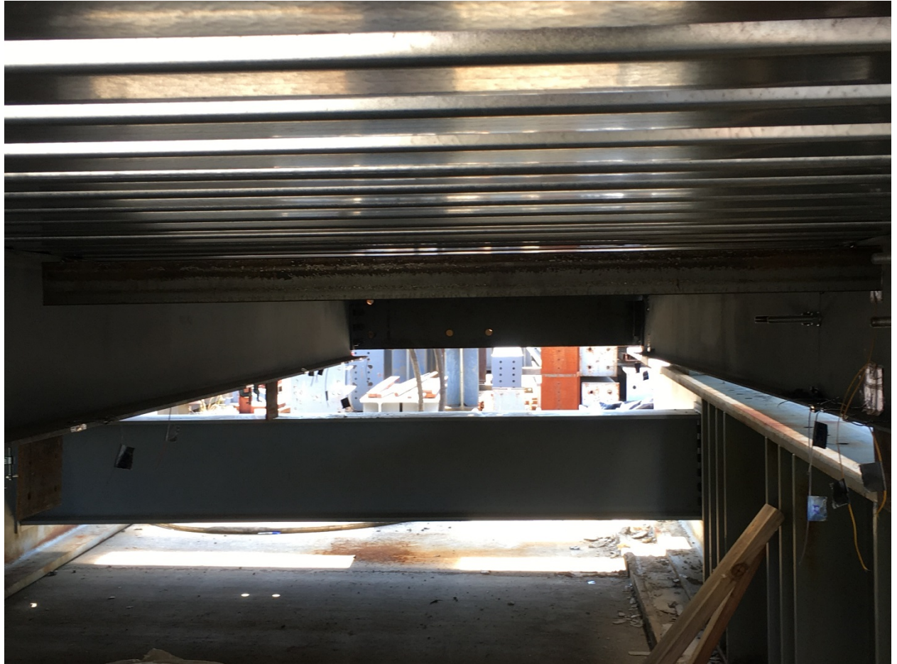
Figure 10: Western bridging on the W12x26 beam.
