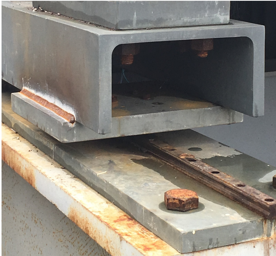
Figure A 7: Northern End Bearing Plate Supporting One End of a W12x106 Beam According to ASCE 7-10 (ASCE, 2013), the minimum acceptable roof slope necessary to preclude considering ponding instability during structural design, assuming free drainage, is \frac{1}{4} " elevation per foot of length. In order to create this slope, 4 steel plates varying in thickness between 1.5 and 2 inches, with a hole pattern identical to that drilled through the webs of the W12x109 members, were placed on the northern coped ends of each beam, such that the holes aligned.
