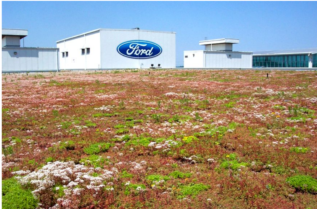
Figure 1: Extensive Ecoroof atop Ford Company's Final Assembly Building in Dearborn, MI. ( http://www.greenroofs.com/projects/pview.php?id=12 )
