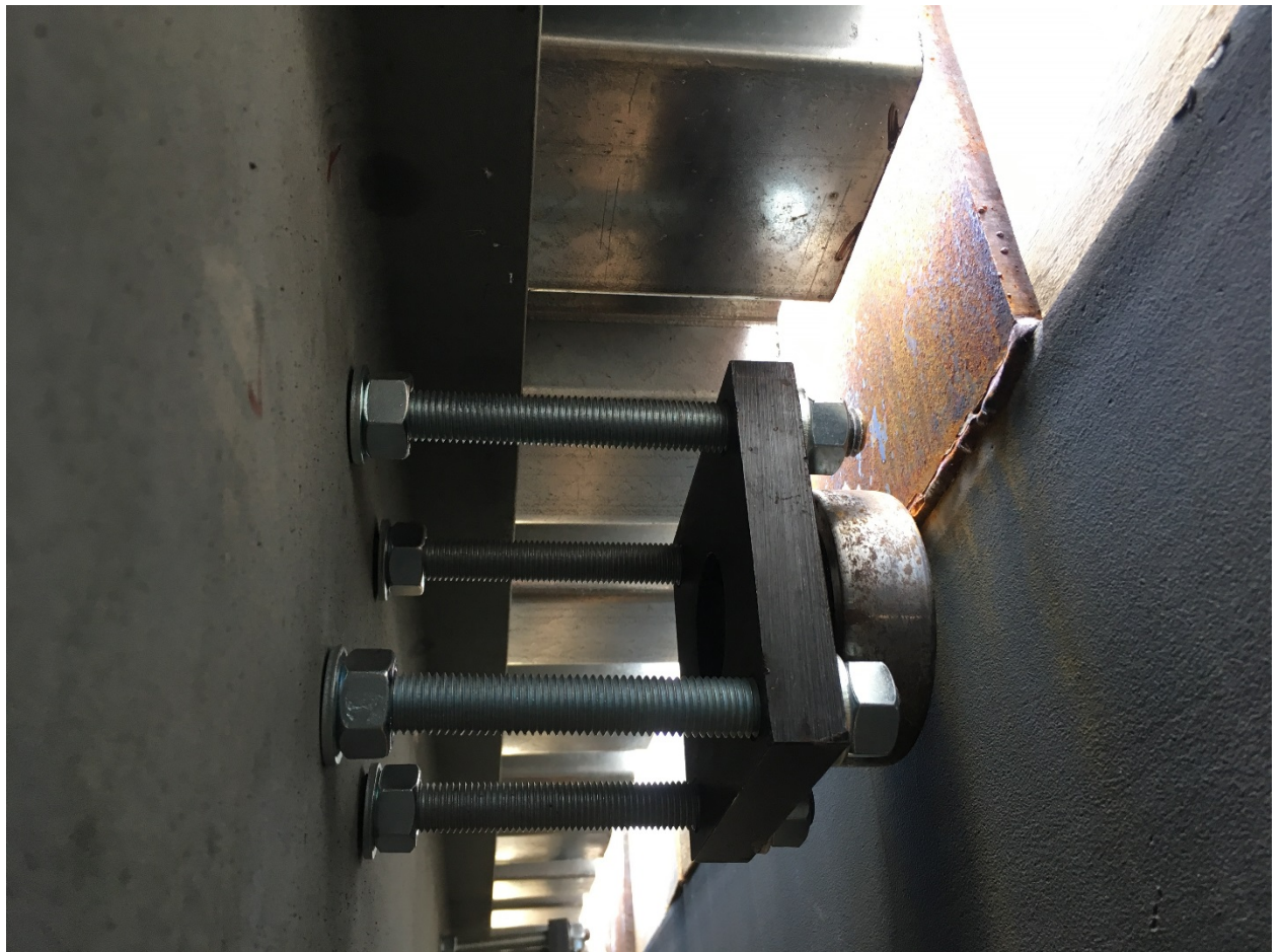
Figure 9: Characteristic Winkel bearing configuration.
