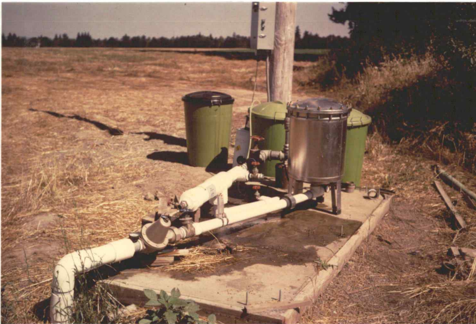
Figure 29. Head of trickle irrigation system.
