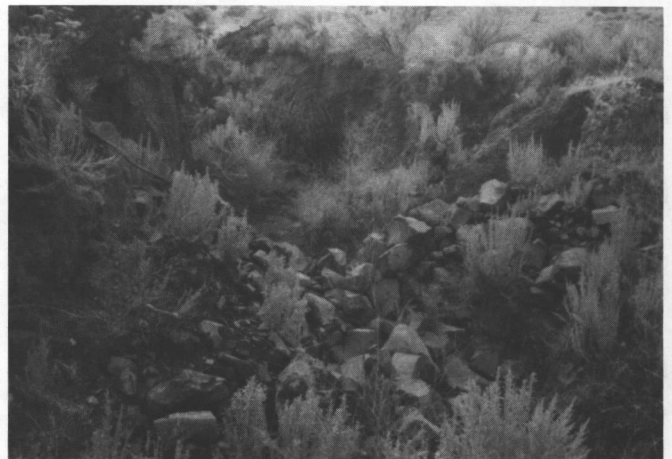
Figure 7-11.—This new structure will allow excess flow to pass over the center. Note the size of the rock.
