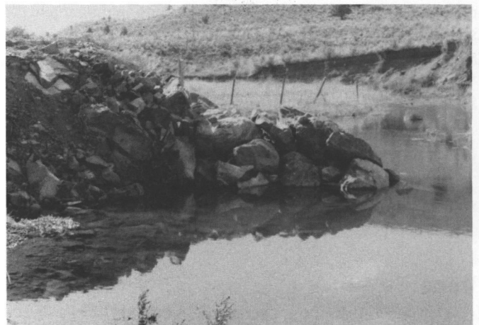
Figure 7-5.—Strength from a large rock is a must to slow water and break or divert its energy.
