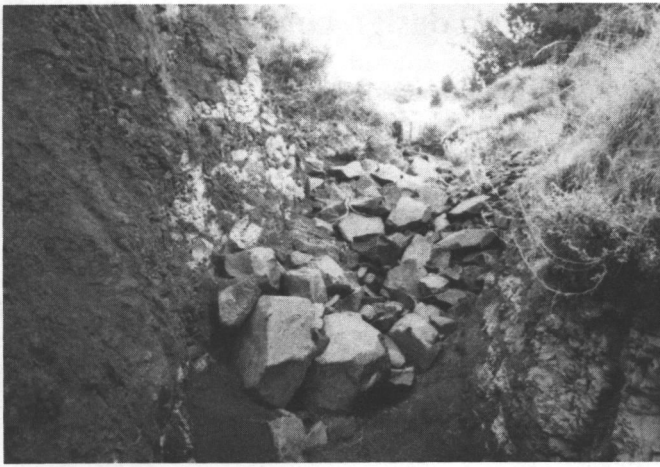
Figure 7-8.—Rock of various sizes will minimize soil movement, to allow vegetation to become established.
