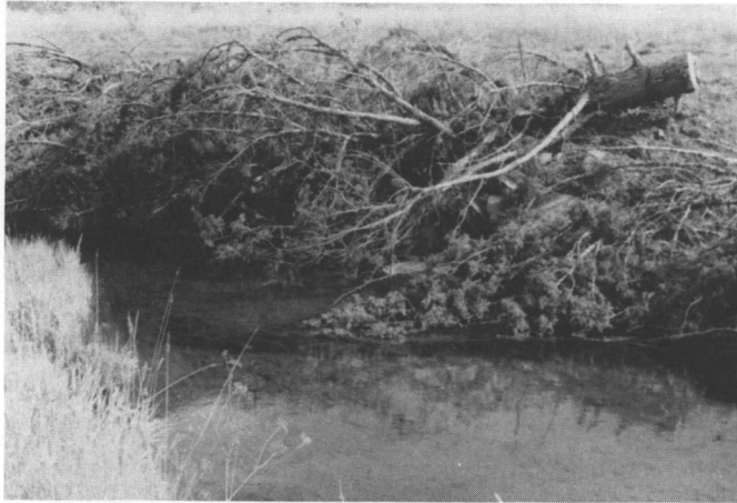
Figure 7-10.—Close contact of the tree trunk and the soil provides the best chance for the bank to become stable.
