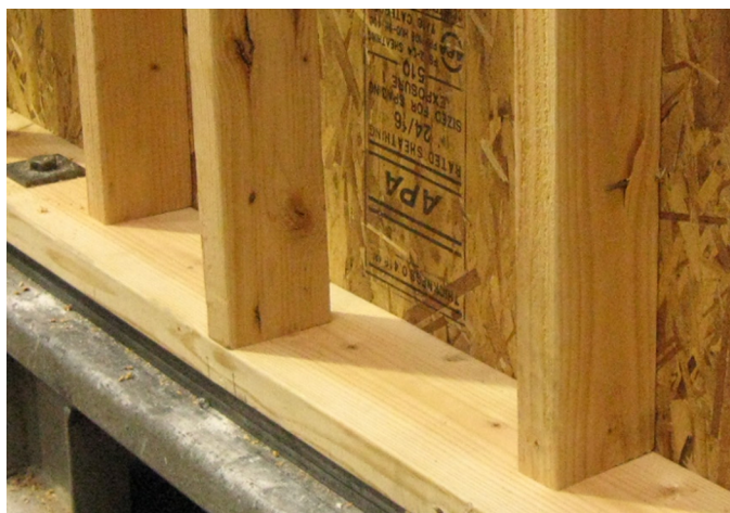
Fig. 1. The 2 × 6 bottom plate and 2 × 4 framing in an SS wall
