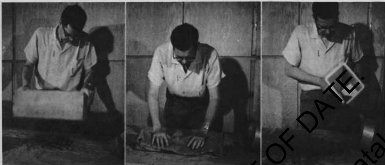
Basic steps in processing dried cones: First shake the cones in a box with a screened bottom; then roll or knead in a burlap bag to remove wings; then pour slowly in front of a fan to separate good seed from hollow seed and chaff.
