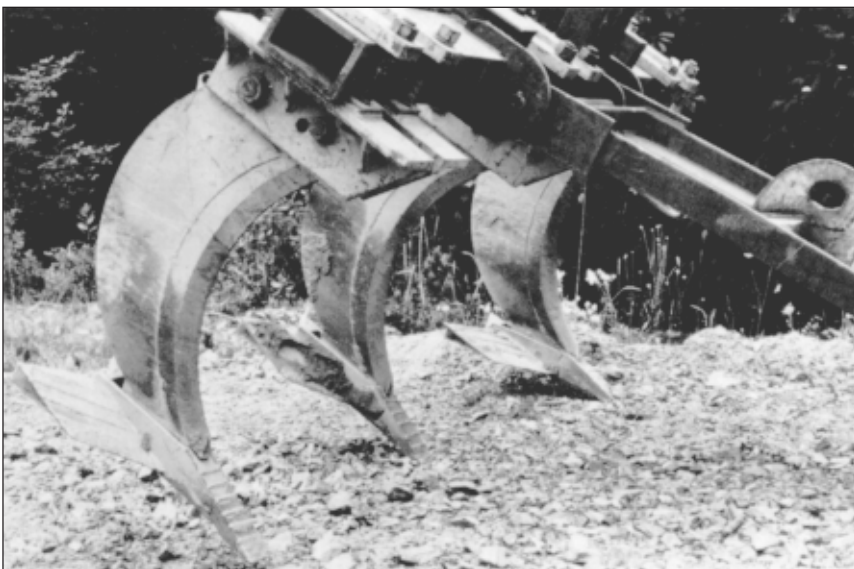
Figure 7.—You can reduce compaction problems after logging by tilling major skid trails and landings with implements like these rear-mounted “winged” ripper teeth.
