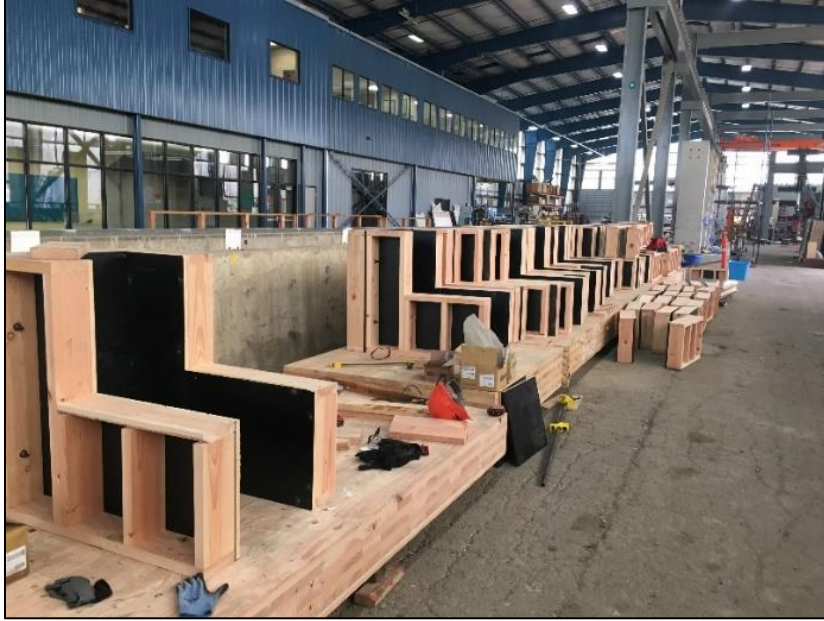
Figure 3.16: Formwork construction.
