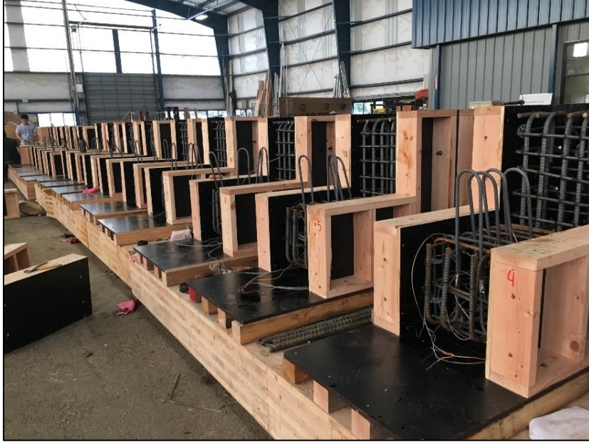
Figure 3.18: Cage is inserted into formwork.
