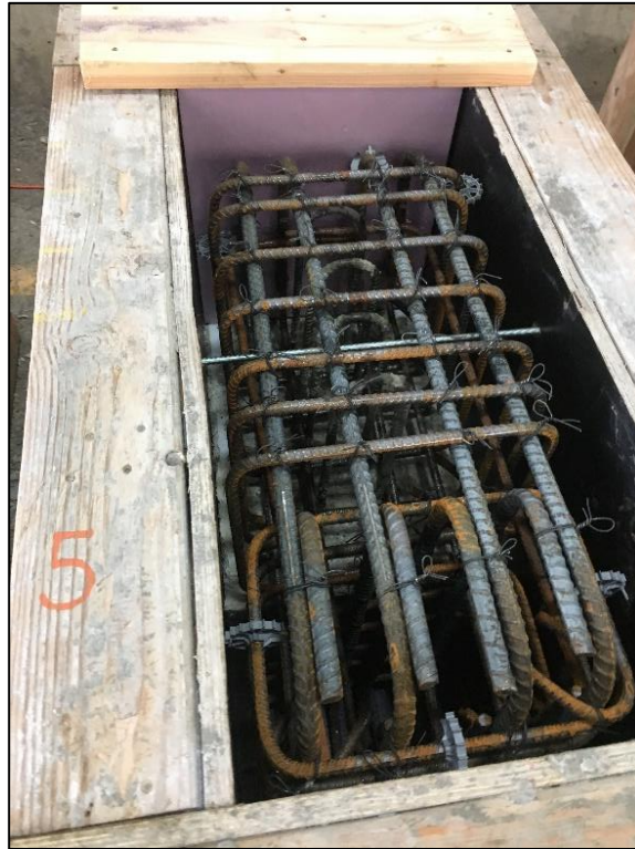
Figure 3.22: Top L-shaped cage placed inside formwork.
