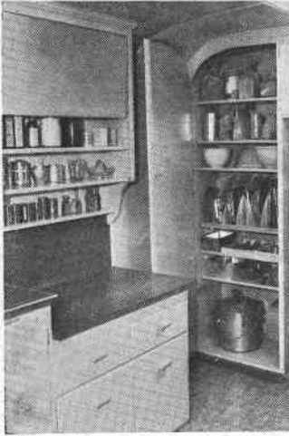
Above: Mixing center. Equipment occupies one shelf of cabinet above mixing table, and five shelves of the floor-to-ceiling cabinet. Note use of slots for flat utensils and shallow boxes for spoons and other small articles.
