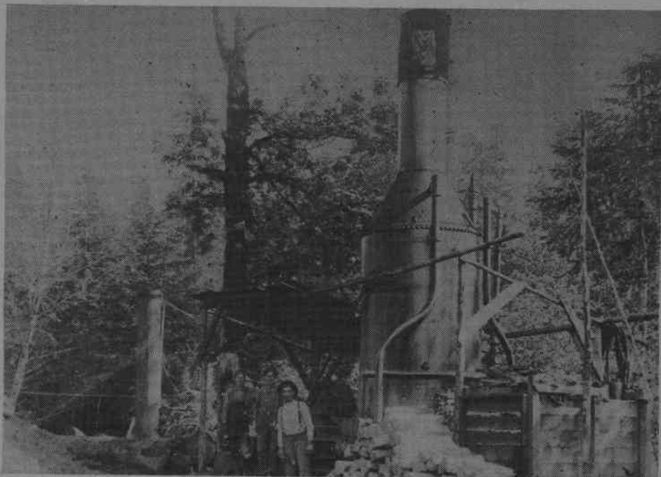
Ca. 1908 Booth Kelley 10x15 Tacoma kicking donkey. Left foreground shows start of chute that went 1400 feet to McKenzie River just above Deerhorn. l-r Geo. Windham, Charlie Carger, Joe Farnum. Louis Polley picture
