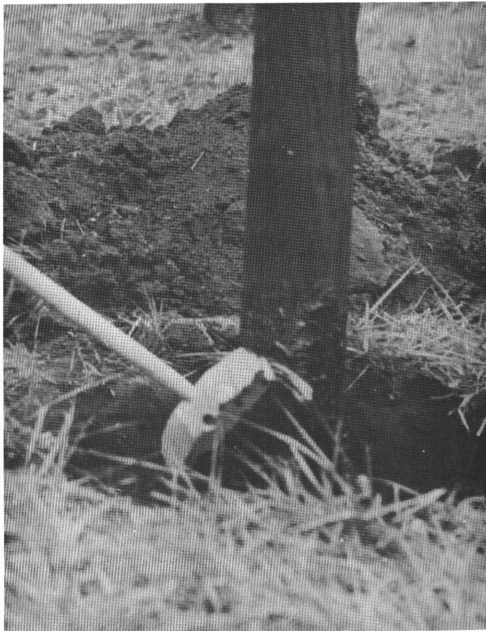
Figure 3.--Fluoride-coal tar paste being applied to a stub with a window brush.
