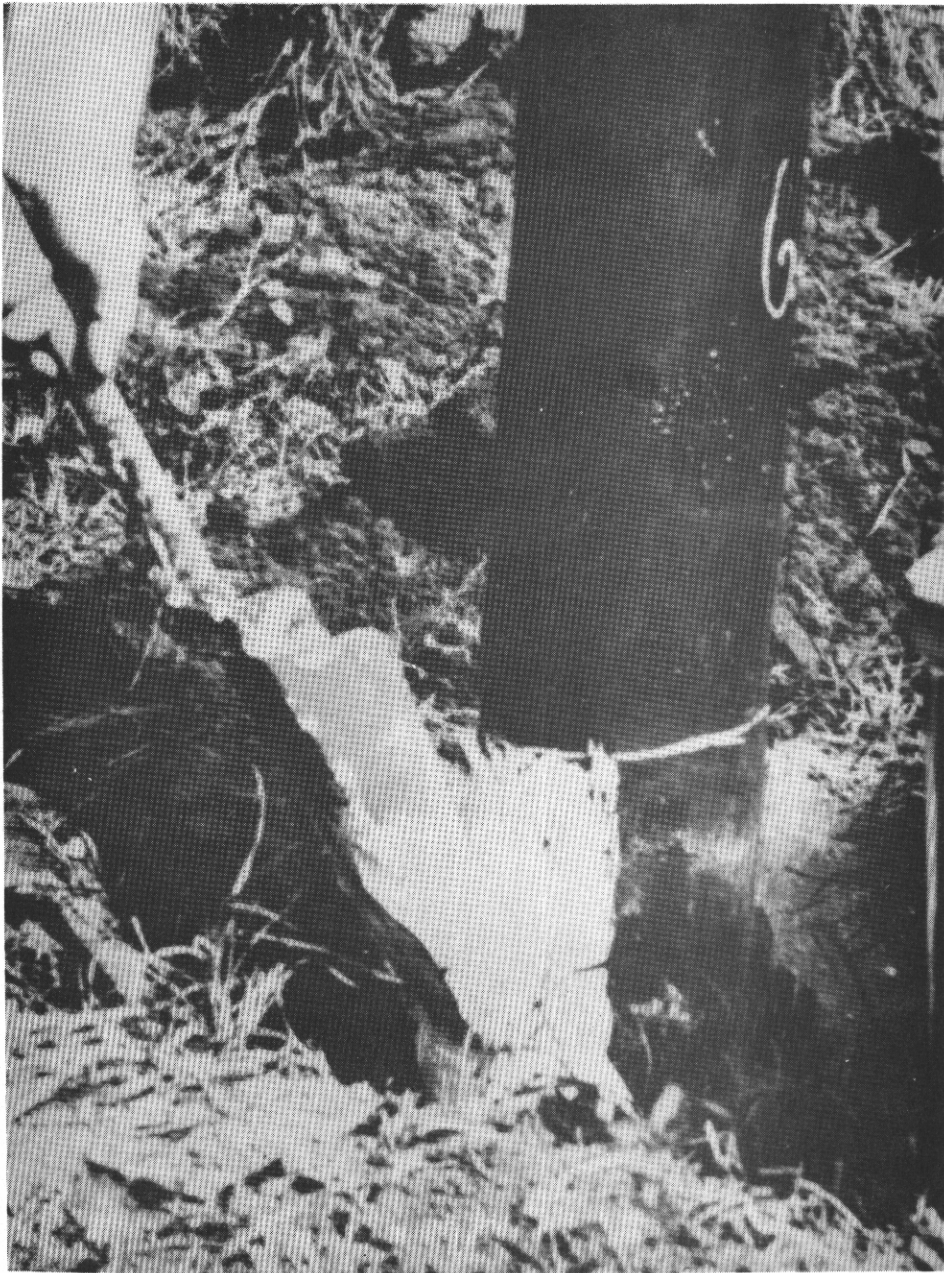
Figure 5. --Scooping penta gel onto a stub.
