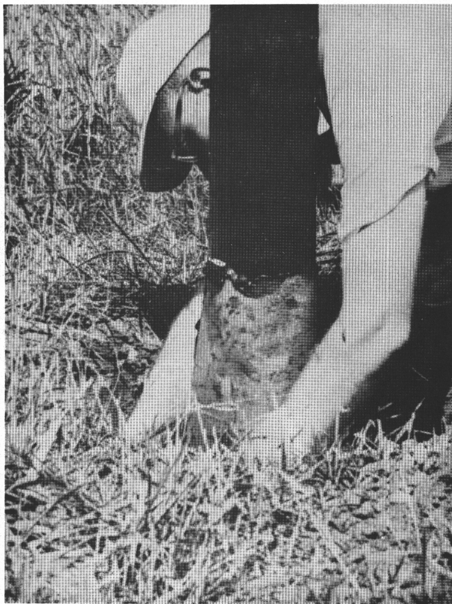
Figure 4. --Wrapping bandage coated with penta grease around pole.
