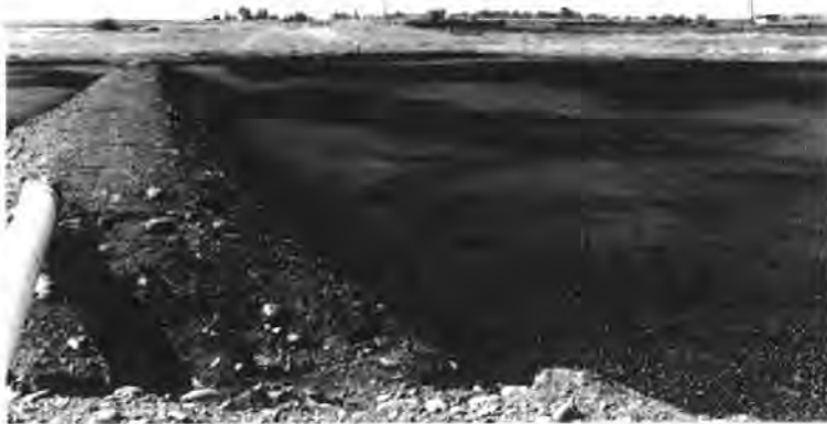
Figure 6. Sludge in drying beds following digestion. Vernon Thorpe Water Quality Control Plant, City of Medford.
