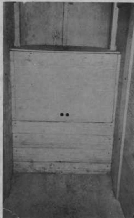
Figure 11. Inside trailer, looking toward ► storage compartment. Door is hinged at top.
