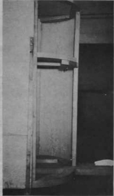
Figure 5. View from side showing ► framing of semi-circular front with one piece of plywood in place.
