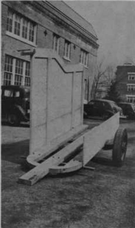
◀ Figure 4. View showing framing of front and side of trailer.
