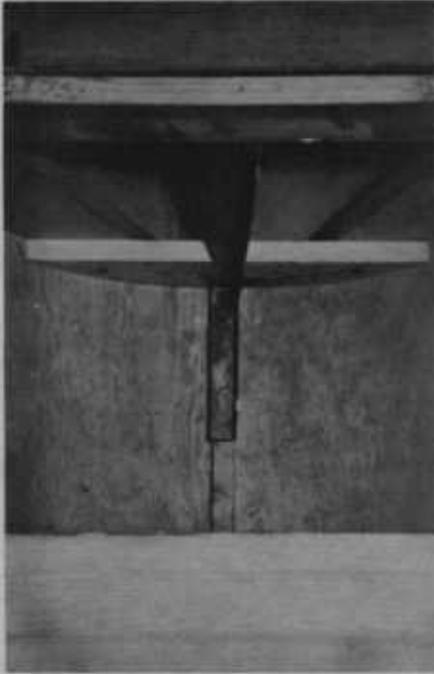
Figure 7. Framing and angle iron brace above storage compartment.
