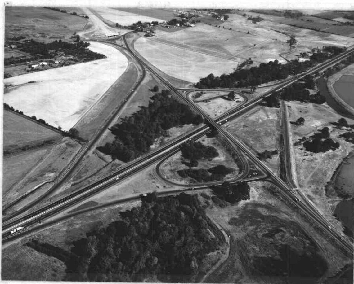
Figure 13. The present North Santiam Interchange exemplifies the semicloverleaf-diamond interchange design. This interchange is designed to handle the heaviest traffic of the four interchange designs examined thus far. The North Santiam Interchange will be expanded to a full cloverleaf in the immediate future. The addition of another semicloverleaf to the present interchange will constitute a full cloverleaf interchange.
