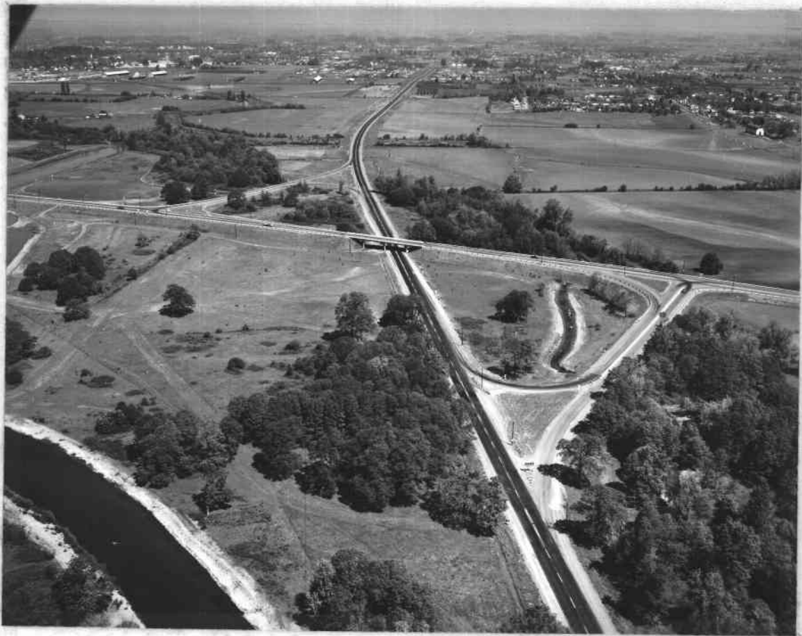
Figure 10. A 1957 view of the North Santiam Interchange, illustrating the semicloverleaf interchange design. Note that this design funnels all traffic on and off the freeway at two locations, one on either side of the overpass.
