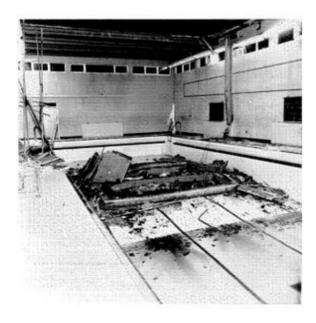
Figure 1-1: John Cass School Roof Beam Collapse [10]
