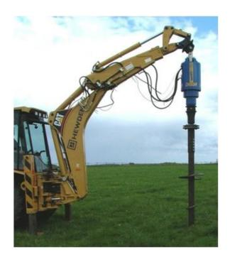
Figure 2.6 Backhoe with torque head installing a helical element (Francis & Lewis International, 2012).
