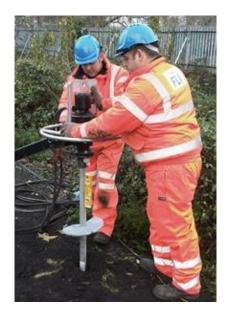
Figure 2.5 Hydraulic hand pack installation of helical anchors (Francis & Lewis International, 2012).
