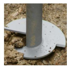
Figure 2.1 Helical plate being torqued into the soil (Magnum Piering, 2012).
