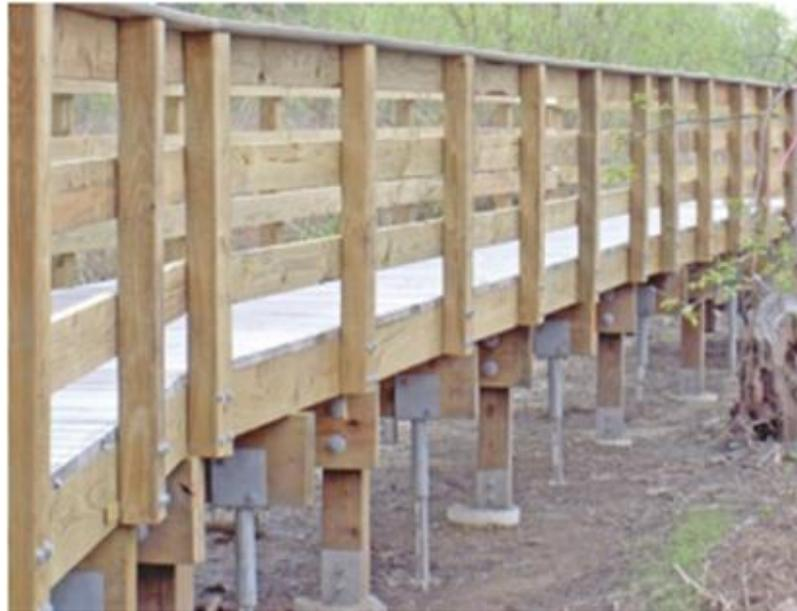
**Figure 2.4 Boardwalk built on helical piles through a marshland. The previous foundation had failed due to settlement; helical piles were used for reconstruction (Hubbel, 2012).**
