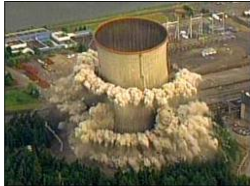
Figure 3: PGE Trojan cooling tower demolition.
