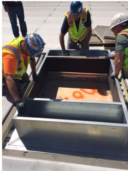
Figure 3.2: Roof curb installation
