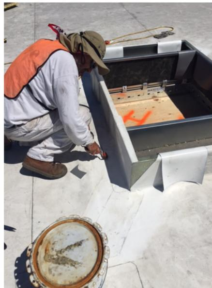
Figure 3.3: Water proofing and insulation installation
