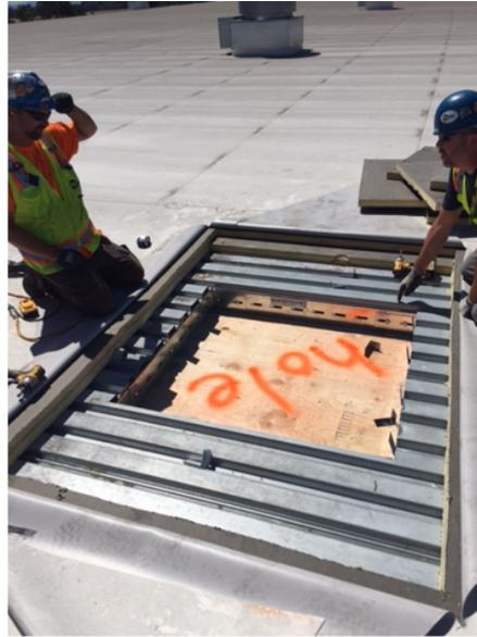
Figure 3.1: Covered roof penetration
