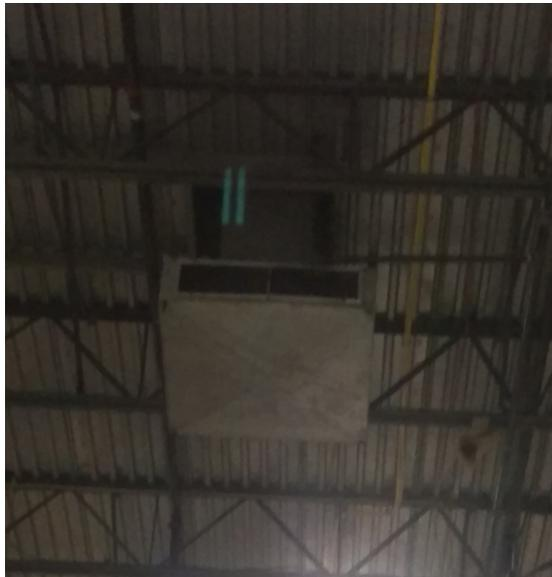
Figure 3.9: MAU heater, interior view
