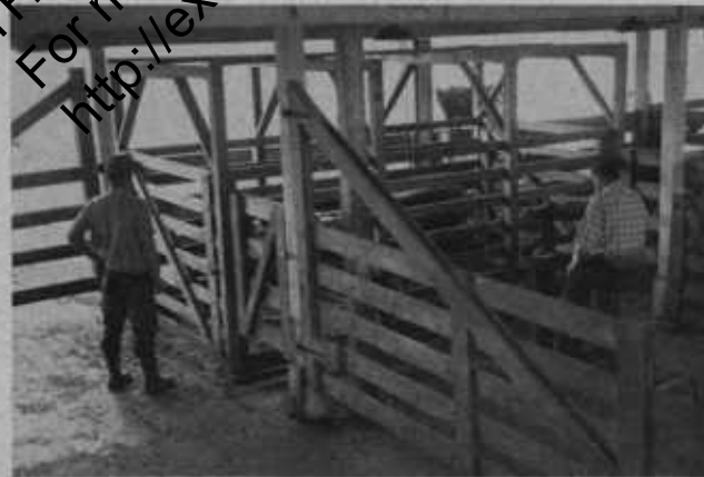
Location of weighman is important. He should be shielded from stock, but in clear view of buyer and seller. He must be able to see the platform and approaches.
