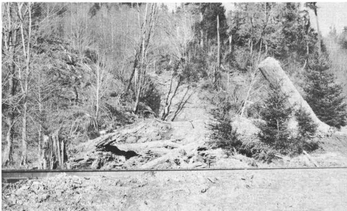
Photo 37.--This tangle of mud, brush, and logging debris was deposited on the railroad in the foreground. Poppino photo NO. 5
