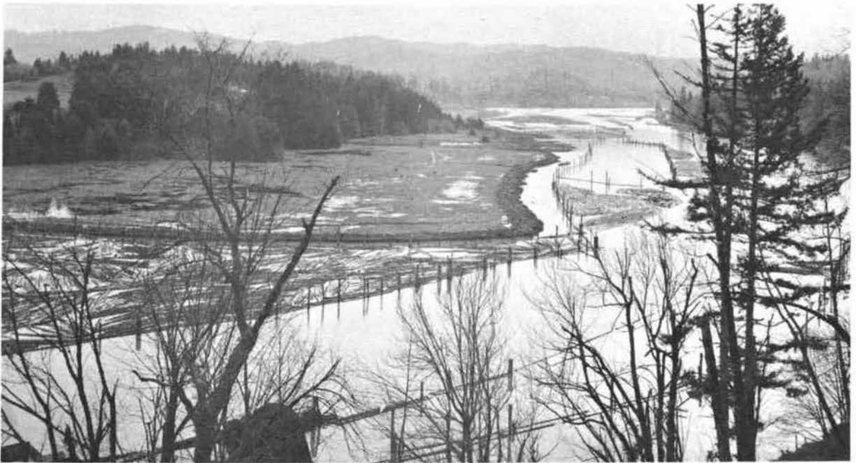
Photo 30.--Pasture on tide lands is often covered with water even when protected by dikes and tide gates. Surface drainage is needed before subsurface drainage can be efficient, Yaquina River, Oregon, 1964. RBSP photo NO. 7-1541-4
