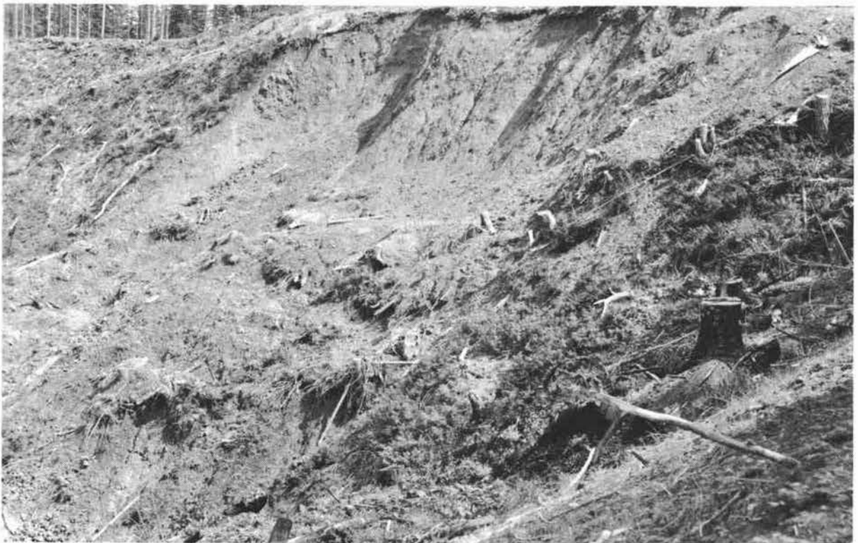
Photo 22.--Slumps or land slides frequently occur after the head-wall portion of a stream is disturbed by roadbuilding. RBSP photo NO. 7-1571-10
