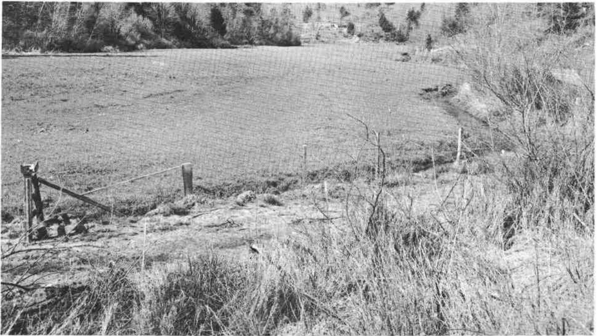
Photo 32.--Sometimes a field can be drained with a well placed interception ditch, Siuslaw S&WCD, Oregon. SCS photo NO. 7-1529-12
