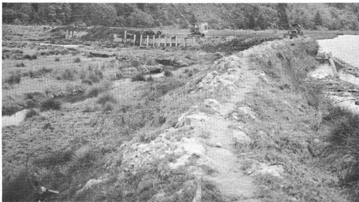
Photo 27.--An inadequate dike and tide gate is being repaired after damage from high water, North Fork Siuslaw River, Oregon, 1963. SCS photo NO. 7-1391-12
