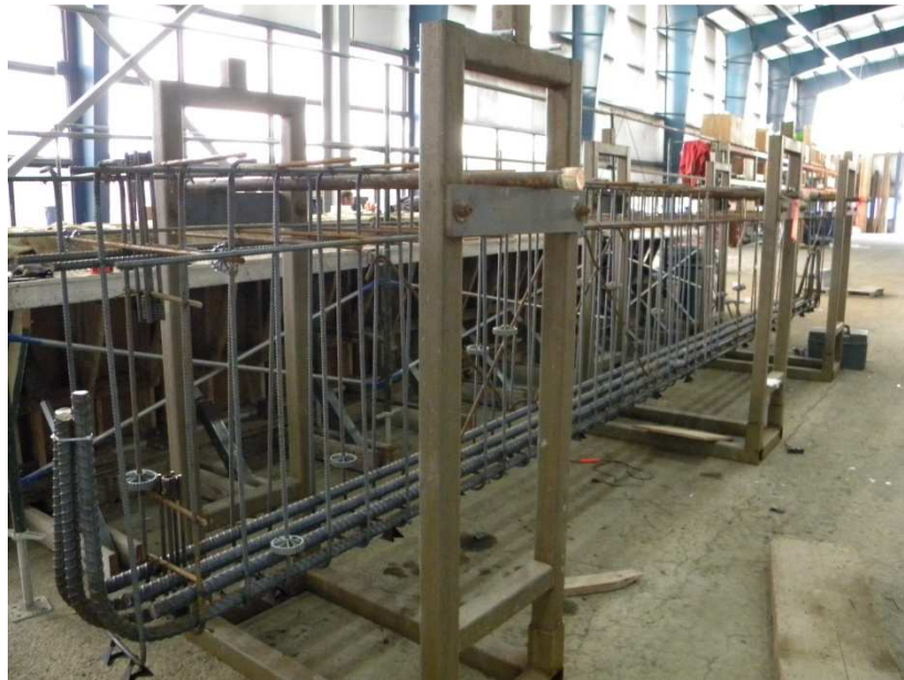
Fig. 5.1 – Example of reinforcing cage
