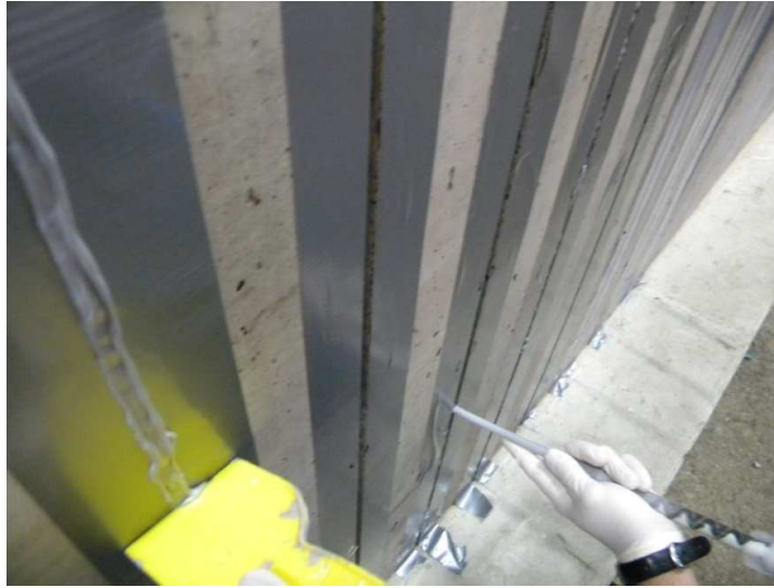
Fig.5.5 – Epoxying CFRP strips into NSM grooves
