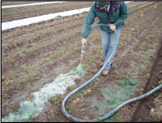
Figure 1. Photograph of hydro-mulch application.
